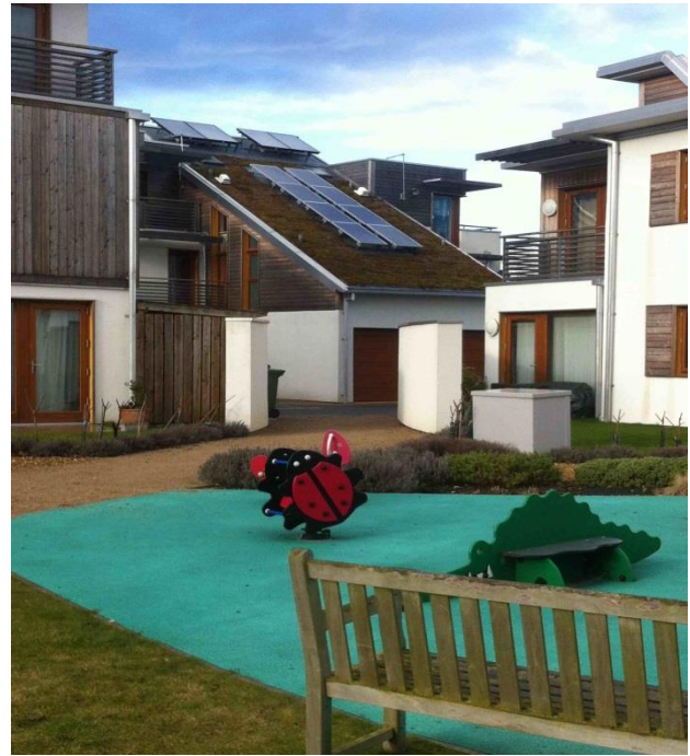
Social and private affordable eco-housing surrounds a communal garden and play area.
