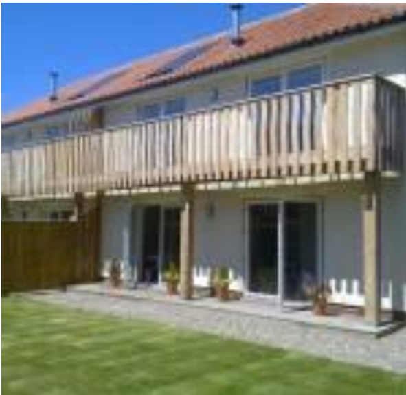
Kesteven council in Lincolnshire built straw-bale houses for about £20,000 less than the same design and scale of project would have cost with brick construction.
